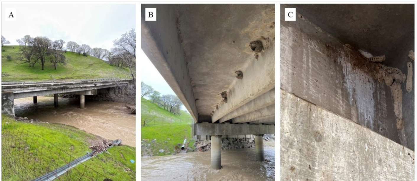
Figure 19. (A) Marsh Creek Bridge - Structure ID 28 C0124. Substructure of structure ID 28 C0124 facility near Marsh Creek Springs, Contra Costa County, California, USA, on Marsh Creek Road over Marsh Creek. (B) Marsh Creek Bridge - Structure ID 28 C0124. Guano staining on the substructure of structure ID 28 C0124 facility near Marsh Creek Springs, Contra Costa County, California, USA, on Marsh Creek Road over Marsh Creek.
