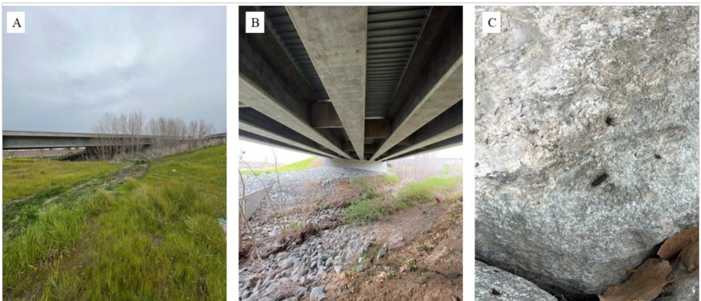
Figure 16. (A) Lafayette Creek Bridge Circa 1915 - No Structure ID. Substructure of a circa 1915 bridge facility near the City of Lafayette, Contra Costa County, California, USA, along El Nido Ranch Road in proximity to Lafayette Reservoir. (B) Lafayette Creek Bridge Circa 1915 - No Structure ID. Guano staining on substructure of a circa 1915 bridge facility near the City of Lafayette, Contra Costa County, California, USA, along El Nido Ranch Road in proximity to Lafayette Reservoir.
