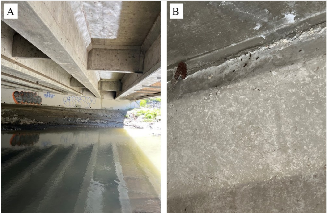
Figure 22. (A) San Ramon Creek Bridge – Structure ID 28 C0087. Substructure of structure ID 28 C0087 facility over San Ramon Creek in Contra Costa County, California, USA. (B) San Ramon Creek Bridge – Structure ID 28 C0087. Substructure of structure ID 28 C0087 facility over San Ramon Creek in Contra Costa County, California, USA, showing guano staining.
