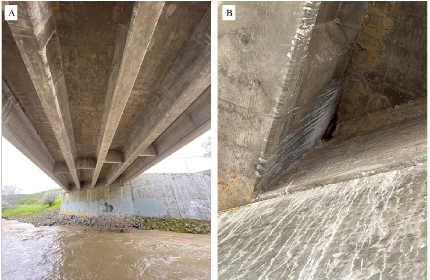
Figure 19. (A) Marsh Creek Bridge - Structure ID 28 C0124. Substructure of structure ID 28 C0124 facility near Marsh Creek Springs, Contra Costa County, California, USA, on Marsh Creek Road over Marsh Creek. (B) Marsh Creek Bridge - Structure ID 28 C0124. Guano staining on the substructure of structure ID 28 C0124 facility near Marsh Creek Springs, Contra Costa County, California, USA, on Marsh Creek Road over Marsh Creek.
