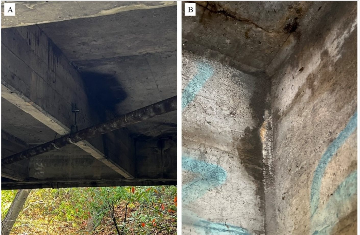
Figure 16. (A) Lafayette Creek Bridge Circa 1915 - No Structure ID. Substructure of a circa 1915 bridge facility near the City of Lafayette, Contra Costa County, California, USA, along El Nido Ranch Road in proximity to Lafayette Reservoir. (B) Lafayette Creek Bridge Circa 1915 - No Structure ID. Guano staining on substructure of a circa 1915 bridge facility near the City of Lafayette, Contra Costa County, California, USA, along El Nido Ranch Road in proximity to Lafayette Reservoir.
