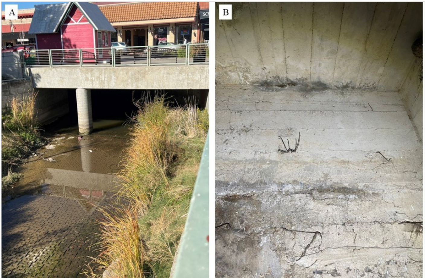
Figure 14. (A) Arroyo del Hombre Bridge – Structure ID 28 C0407. Superstructure of structure ID 28 C0407 facility in downtown Martinez, Contra Costa County, California, USA, along Arroyo del Hombre Creek. (B) Arroyo del Hombre Bridge – Structure ID 28 C0407. Substructure of structure ID 28 C0407 facility in downtown Martinez, Contra Costa County, California, USA, along Arroyo del Hombre Creek. Guano staining.
