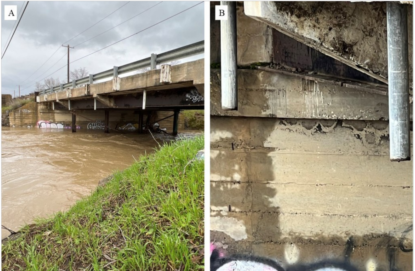
Figure 18. (A) Marsh Creek Structure ID – 28 C0145. Superstructure of structure ID 28 C0145 facilities near the City of Brentwood, Contra Costa County, California, USA, on Marsh Creek Road over Marsh Creek. This facility has been replaced since the field survey occurred. (B) Marsh Creek Structure ID – 28 C0145. Guano staining on the superstructure of structure ID 28 C0145 facility near the City of Brentwood, Contra Costa County, California, USA, on Marsh Creek Road over Marsh Creek.
